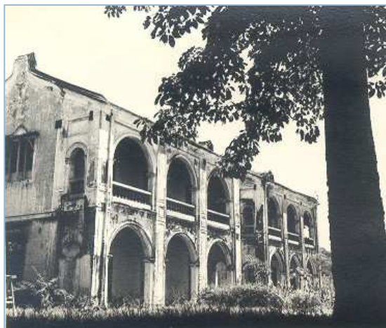
Private Ward Block, Swatow Mission Hospital (PCE/FMC I Additional/109)
