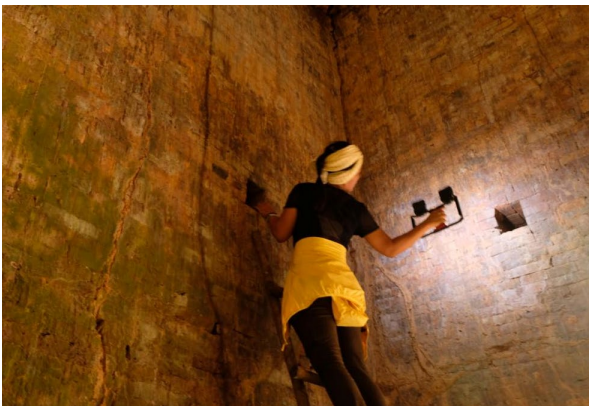
Observing holes from deteriorated hooks on the wall of Damrei Krab temple on Phnom Kulen
