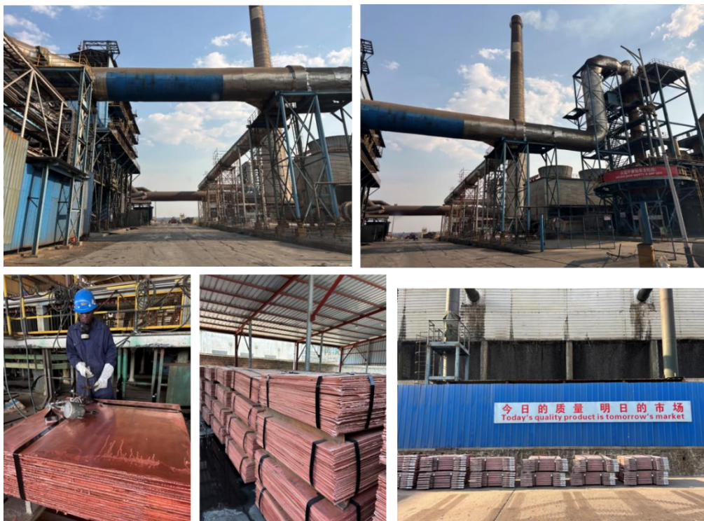
Figure 8. Copper refining in Zambia. Source: photos were taken in the Chambishi copper smelter in Zambia
