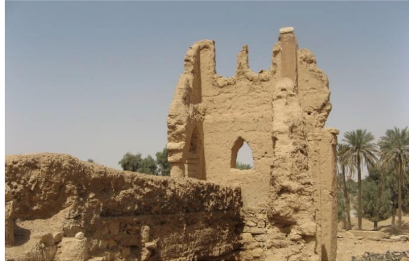
Figure 7: Remains of the bridge leading from Unit 2 to Muhammad bin Sa'ud (Al-Mughnam, 2016).
